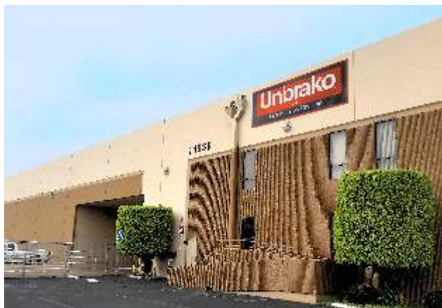
West Coast Distribution Center
